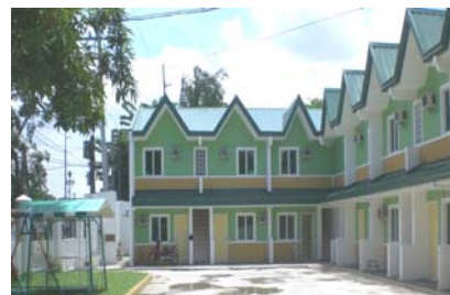
Repair of 10-door apartment at Malacanang, Manila
