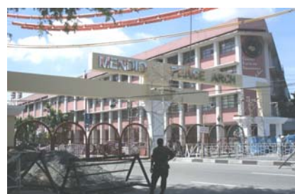
Construction of Peace Arch at Mendiola, Manila
