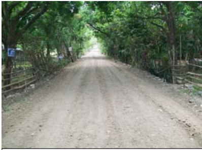
Construction of F-M-R at Brgy Cayabu, Tanay, Rizal
