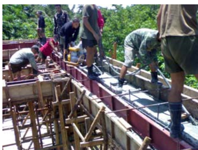
Construction of NADESCOM Building, CGEA, GHQ
