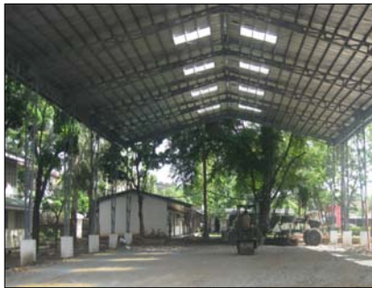
Construction of Covered Court at Camp Atienza, Libis, QC
