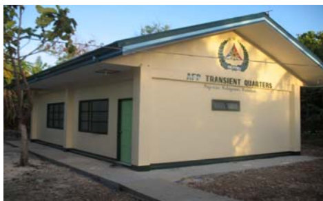
Construction of Transient Facilities at Pag-asa, Island Palawan
