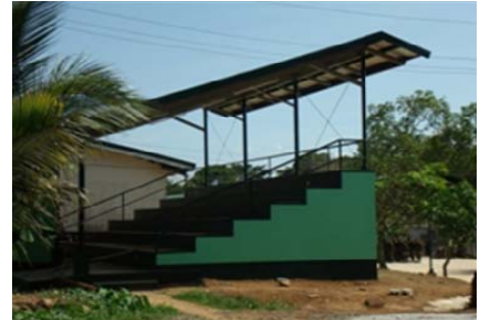
Construction of Bleacher Nr 1 at Camp Capinpin, Tanay, Rizal
