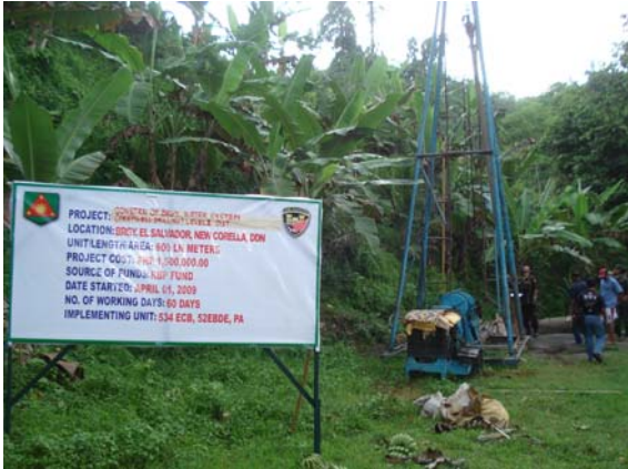
Construction of Water System (Deepwell Drilling Level II)
