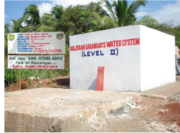
KBP Water System
