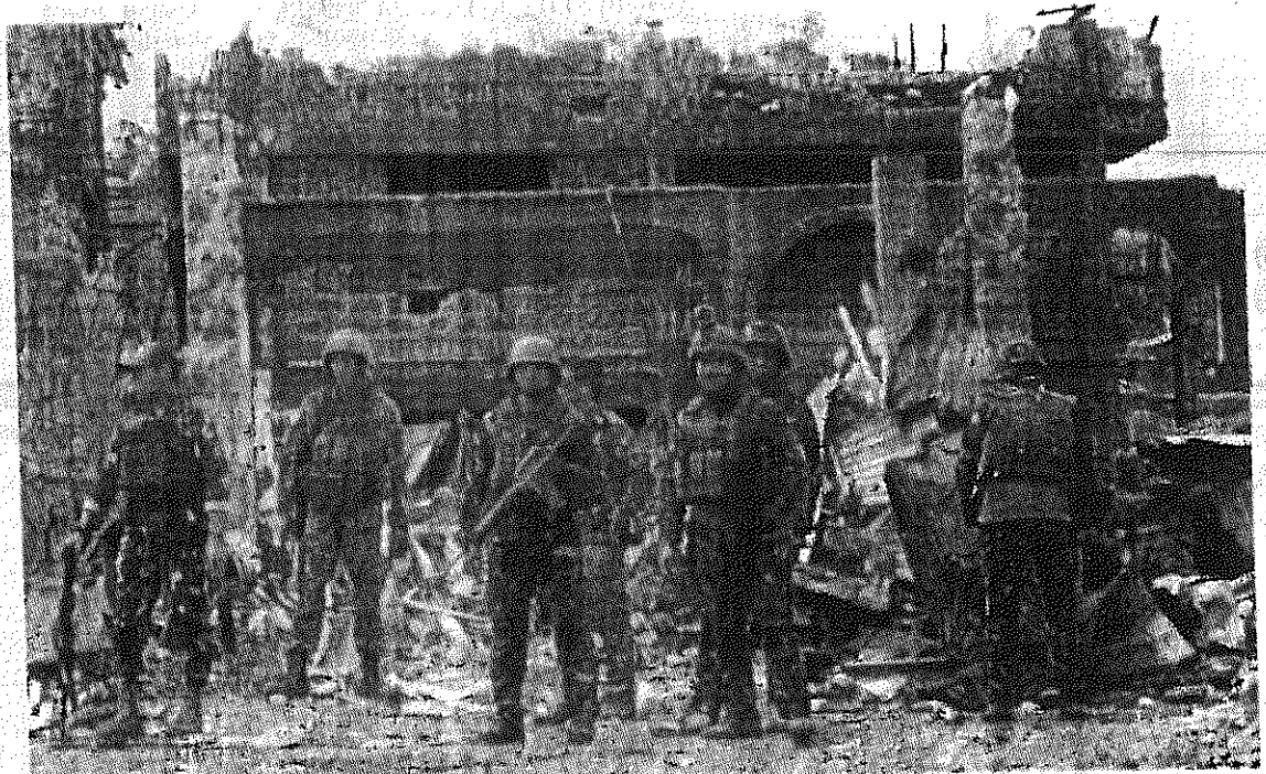
Soldiers on the front line in Marawi City (PDI photo)
