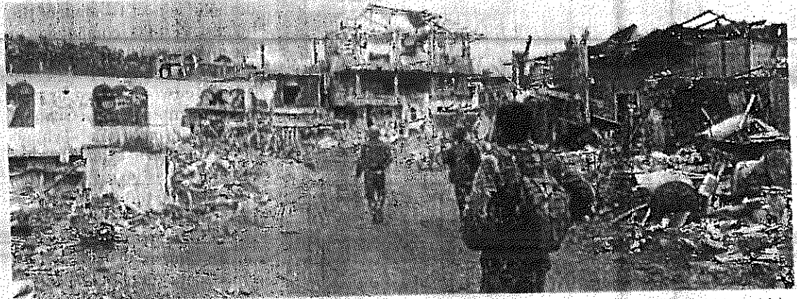
The Marawi siege destroyed houses, schools and other buildings, reducing much of Marawi to rubble.
