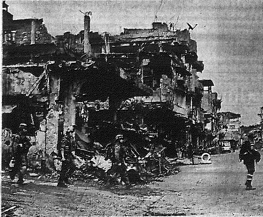
FROM THE RUBBLE – Soldiers go on patrol amid heavily damaged buildings and houses in Marawi City, as government forces continued their assault against pro-Islamic State (IS) militants. (Reuters)
