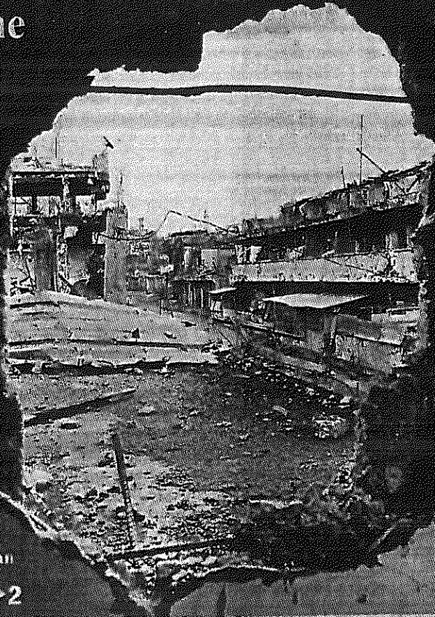
A DEVASTATED CITY – A hole in the wall of a building gouged by an artillery or rocket round offers a view of the extensive damage in Marawi City after more than 100 days of fighting. (Romeo Ranoco/Reuters)
